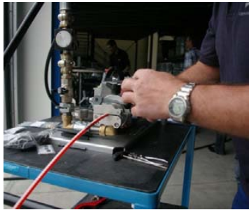
Micro-duct air tightness inspection
