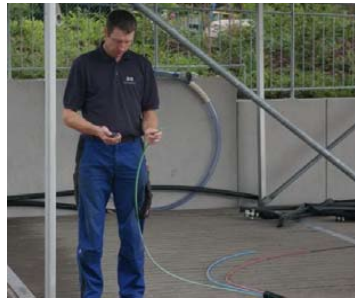
Clean the Micro-duct
